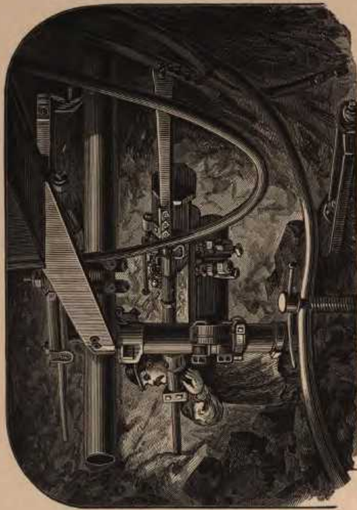
West Heading, with Burleigh Drill, from Photograph taken with Magnesium Lights.
