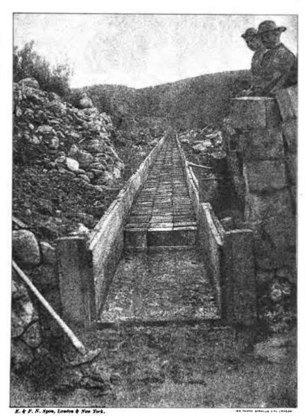
SLUICE. Showing how the false bottom of blocks is put in:
