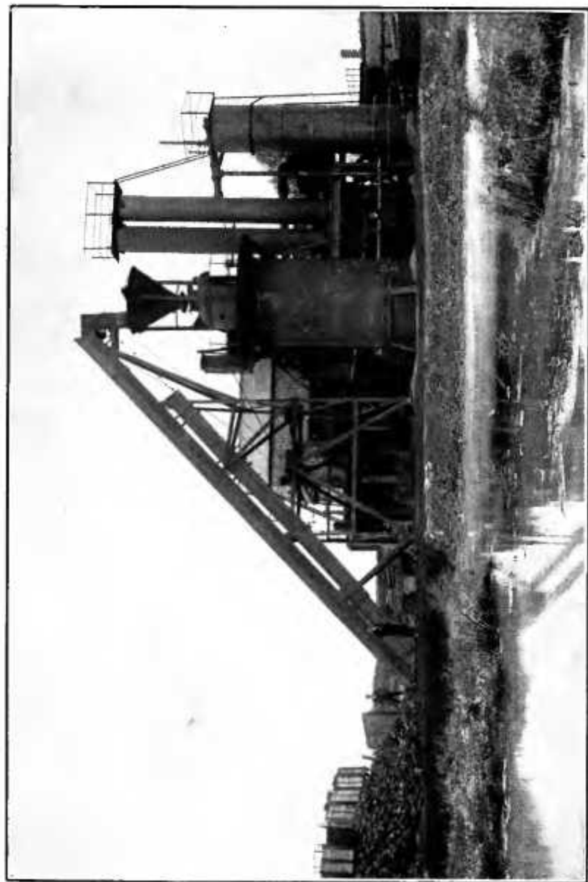
The first producer plant in the world making regularly sulphate of ammonia and producer gas from wet peat.
