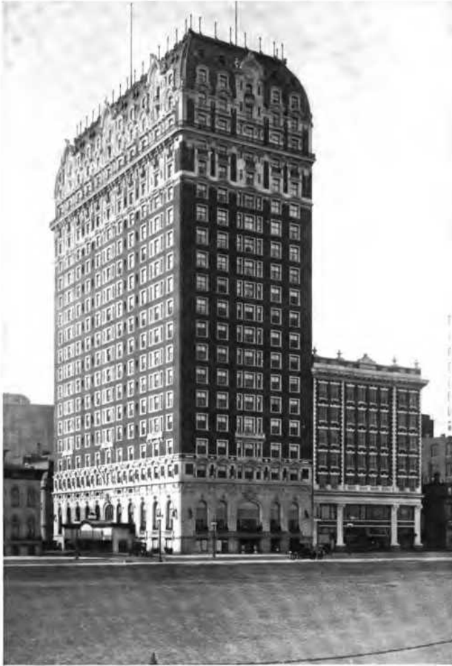
BLACKSTONE HOTEL, CHICAGO, ILL., OPERATING 1012 HORSE-POWER OF STIRLING BOILERS
