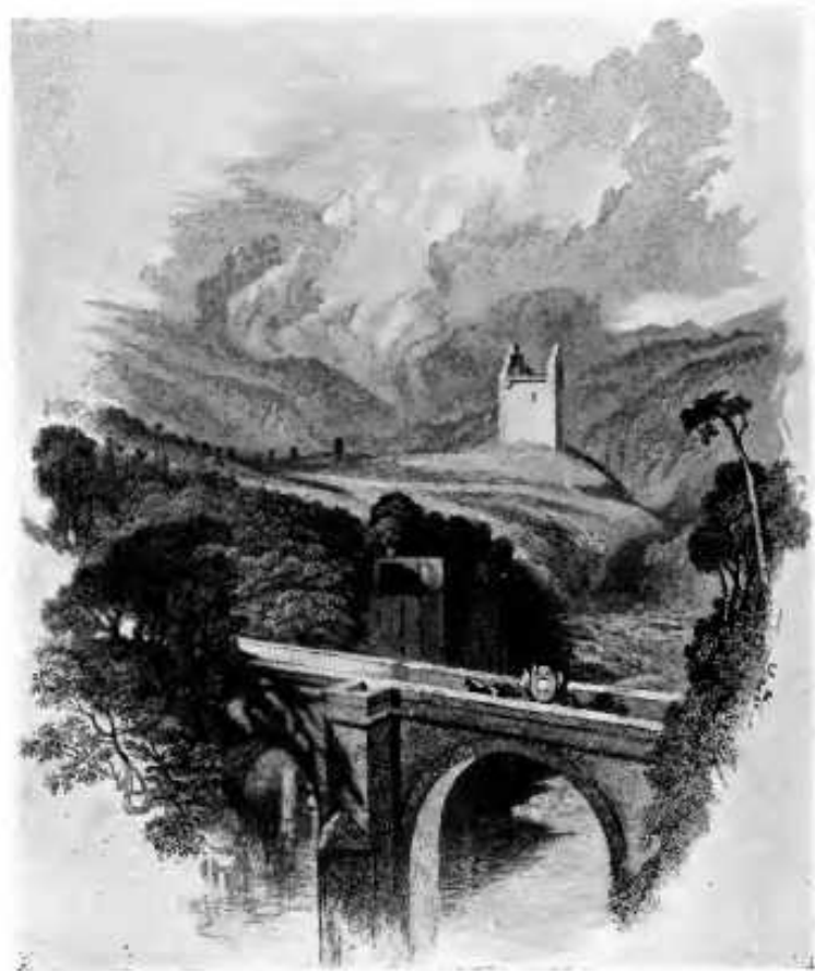
GILNOCKIE TOWER AND HOLLOW'S BRIDGE
