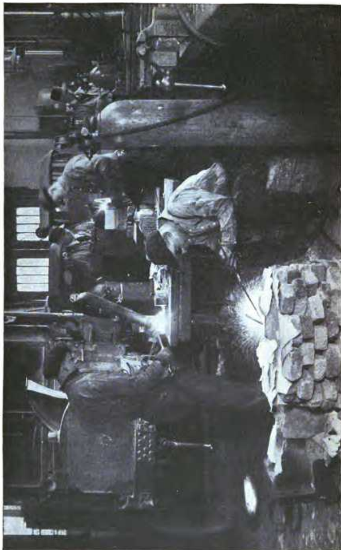
OXY-ACETYLENE WELDING IN AN AUTOMOBILE REPAIR SHOP
