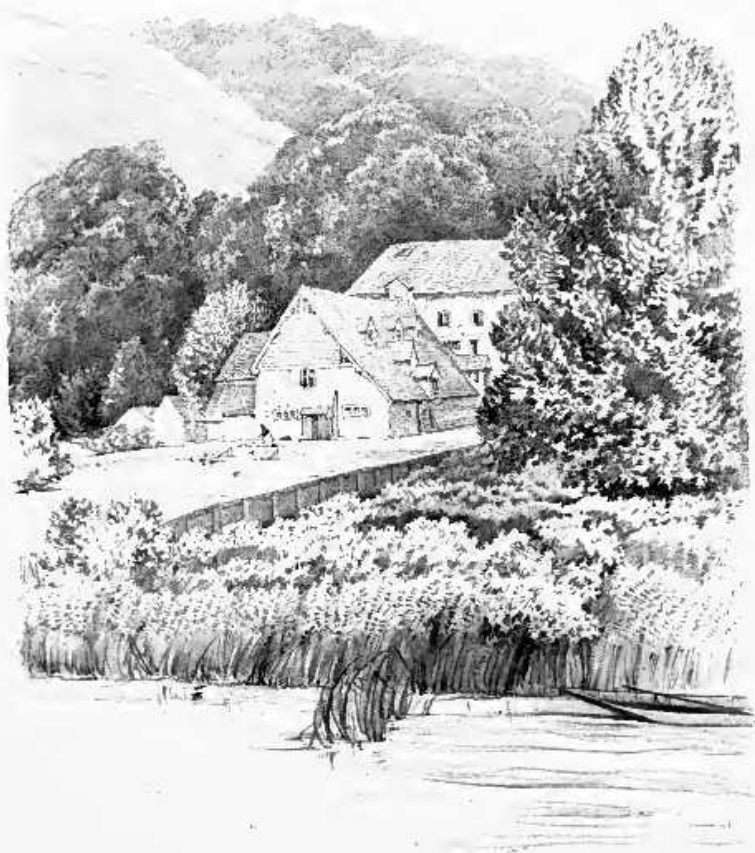
1. STREATLEY MILL, BERKSHIRE.
