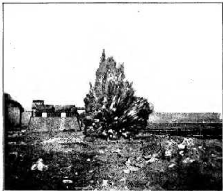
Blasting a Test Hole.
