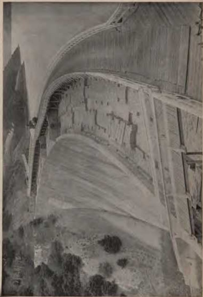
THE TOP OF CENTRAL SPRINGS DAM—SHOWING THE METHOD OF BLOCKING.
