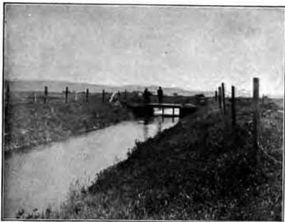
IRRIGATION DITCH, FORT HOMIE.
