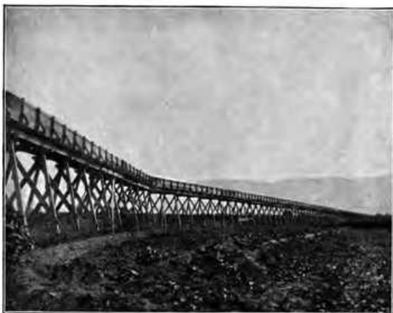
IRRIGATION FLUME, FORT HOMIE.
