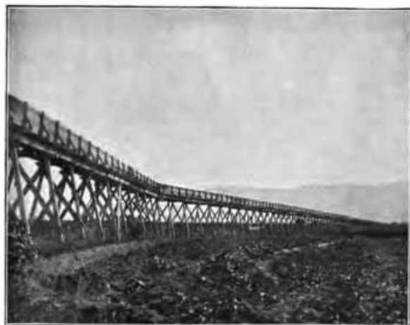
IRRIGATION FLUME, FORT ROMIE.
