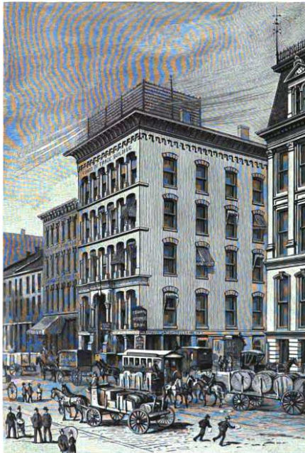
LOUISVILLE BOARD OF TRADE BUILDING.
