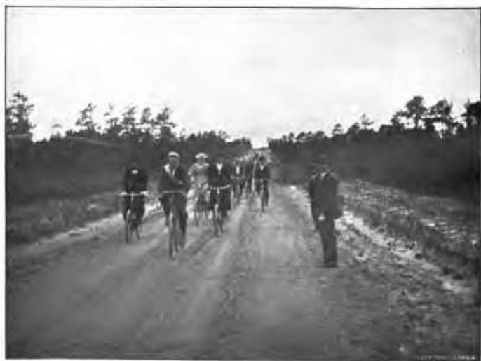
Hammonton and Absecon Road, Camden Co. After Improvement.
