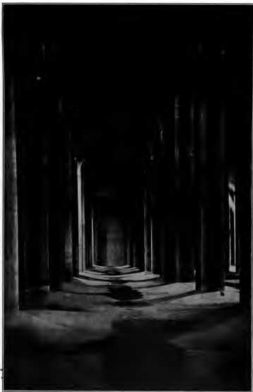
Interior of covered pure-water reservoir at Washington, D. C., before being filled with water. It is covered for the purpose of keeping the filtered water clean.
