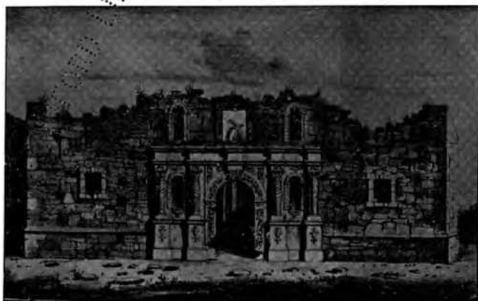
THE RUINS OF THE ALAMO—1838-49. EXTERIOR VIEW.
