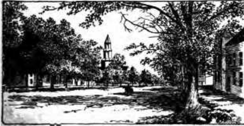
DUKE OF GLOUCESTER STREET, COMING WEST.
