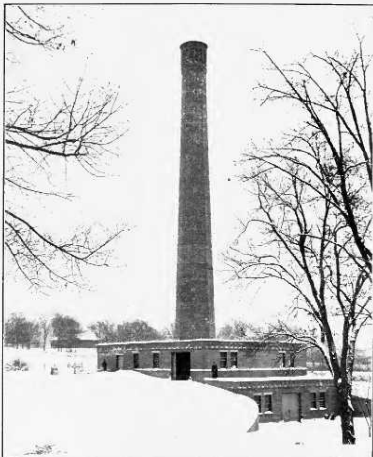
Crematory built by The Municipal Engineering Company at Fort Leavenworth, Kans.
