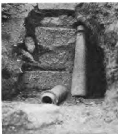
Hard Burned Clay Sewer Pipe laid in Island of Crete 5000 B. C. and still in perfect condition. —Courtesy Clay Products Association
