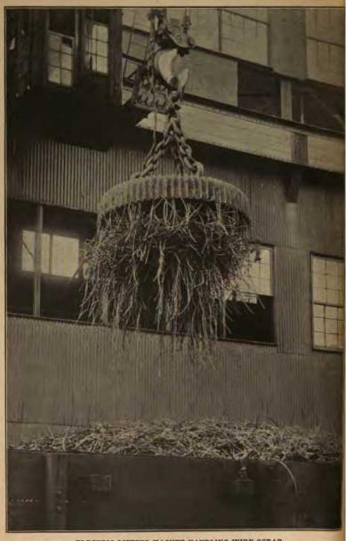
ELECTRIC-LIFTING MAGNET HANDLING WIRE SCRAP
