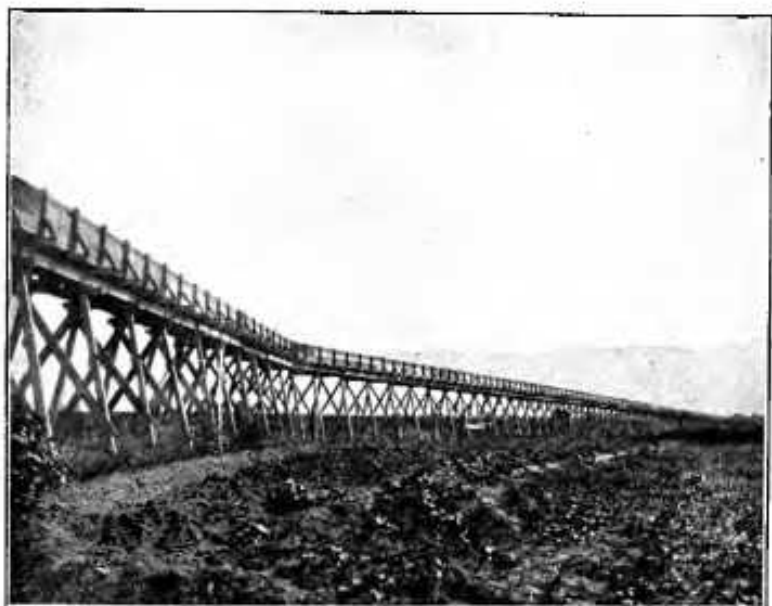
IRRIGATION FLUME, FORT ROMIE.
