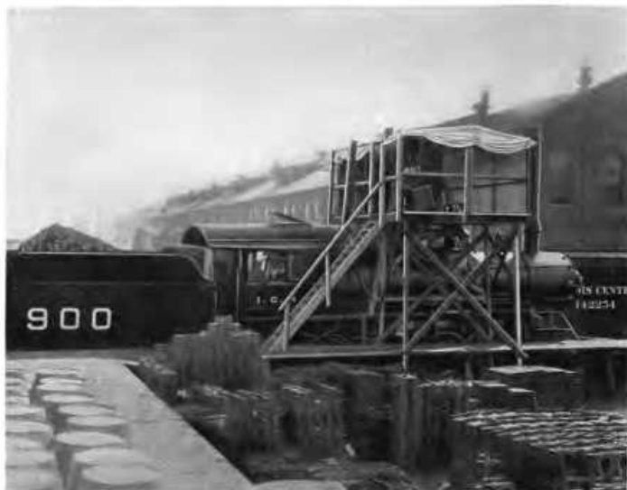
LIFT APPARATUS AS ERECTED FOR LOCOMOTIVE TESTING AT BURNSIDE, ILLINOIS
