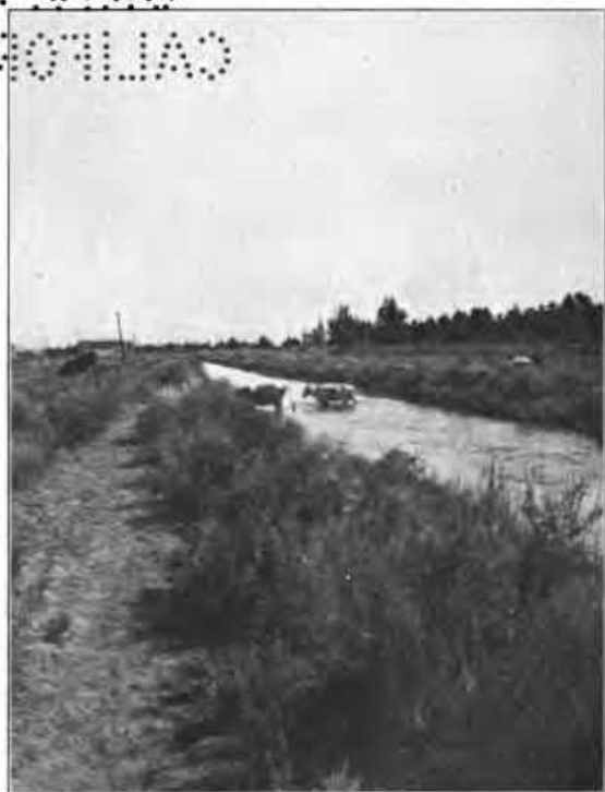
PILOT BUTTE CANAL NEAR REDMOND
