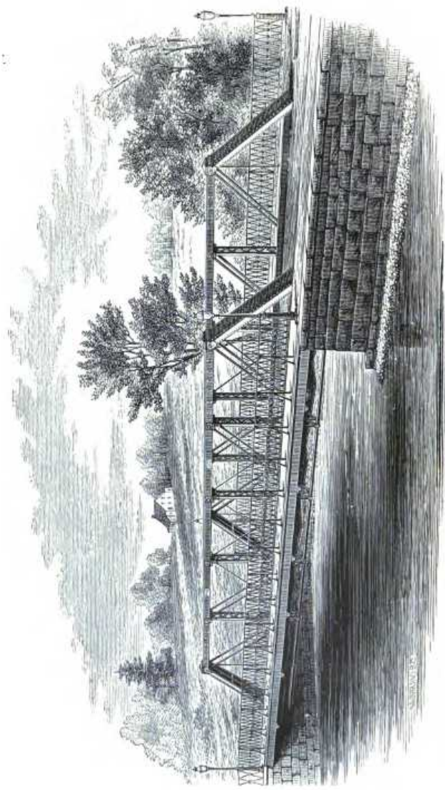
BRIDGE AT PLAINFIELD, N. J. BY THE AUTHOR. 104 FEET SPAN ; 25 FEET ROADWAY ; 8 FEET SIDEWALKS ; 100 POUNDS PER SQUARE FOOT ; FACTOR OF 5 FOR SAFETY.
