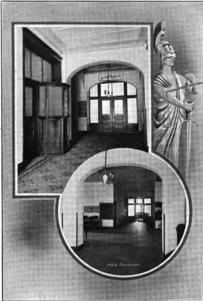
Main Vestibule and Corridor of Law Department.
