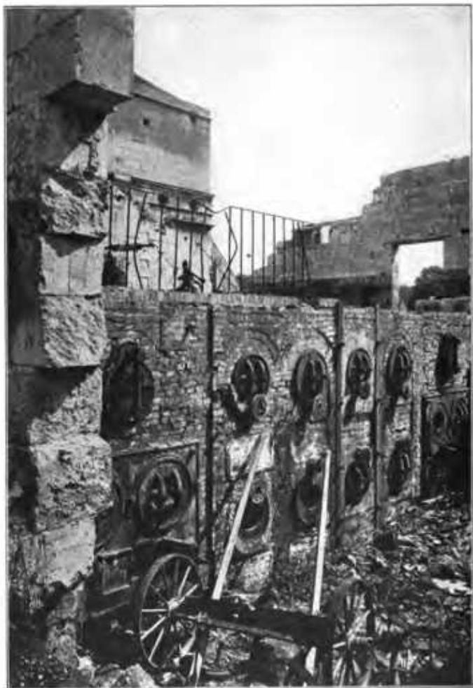
German thefts of factory equipment in northern France. Boiler-room in a factory at Chiry-Ourscamp, Oise.
