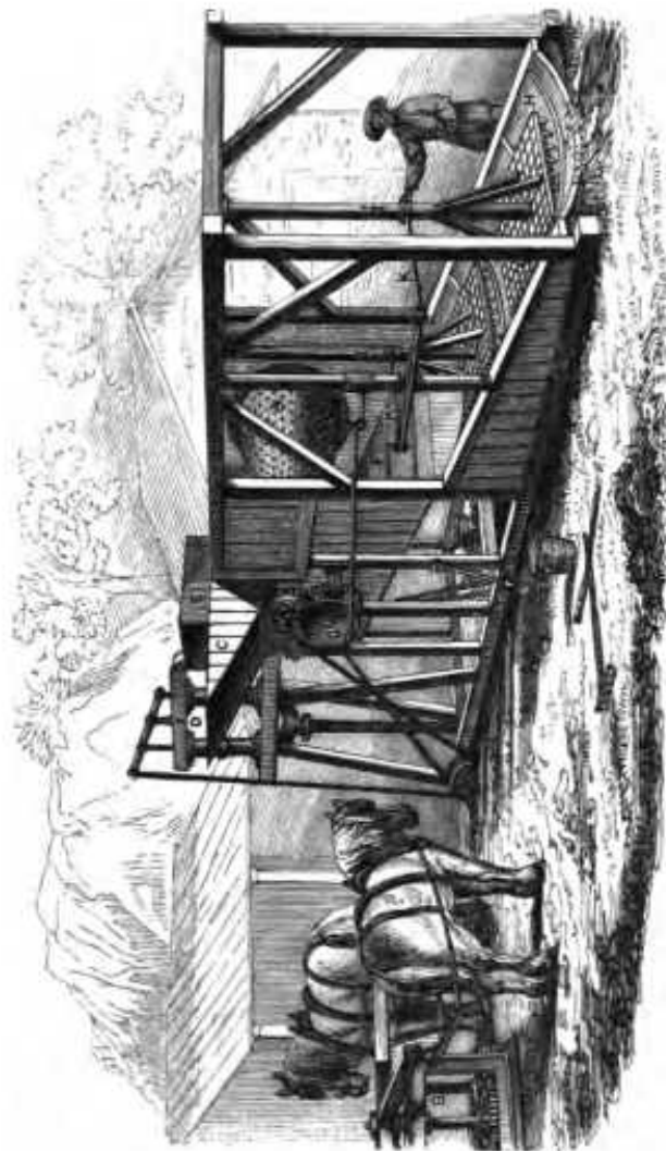
GOLD-WASHING APPARATUS EMPLOYED IN THE URAL.
