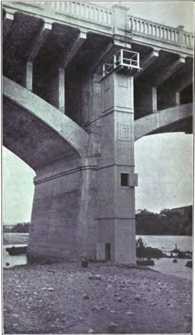
Automatic Water Stage Recorder installed on Highway bridge across the Colorado River at Congress Avenue, Austin, Texas, maintained by the Board of Water Engineers of Texas, the United States Geological Survey cooperating.
