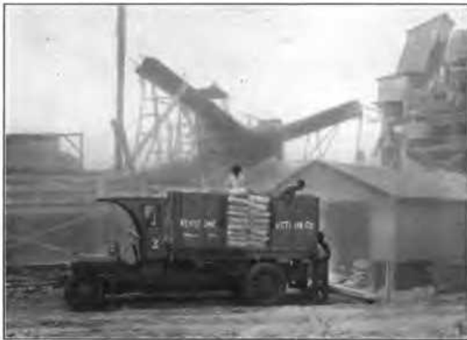
Illustration of the use of a motor-truck in contracting engineering work. This particular truck, according to its owners, did the work of 10 two-horse teams in hauling sack cement to be used in the construction of the great Catskill Aqueduct, New York City
