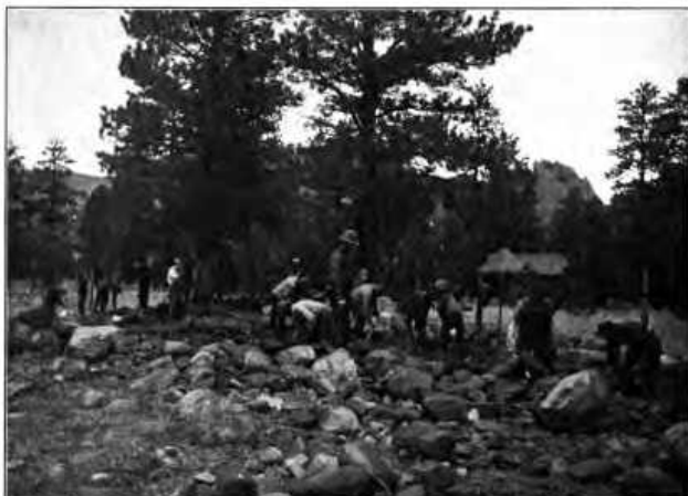
Pioneer Work on Stonewall Road, Near Trinidad. Mr. Radford's Cottage in Right Background. Work Prosecuted Under Supervision of Committee
