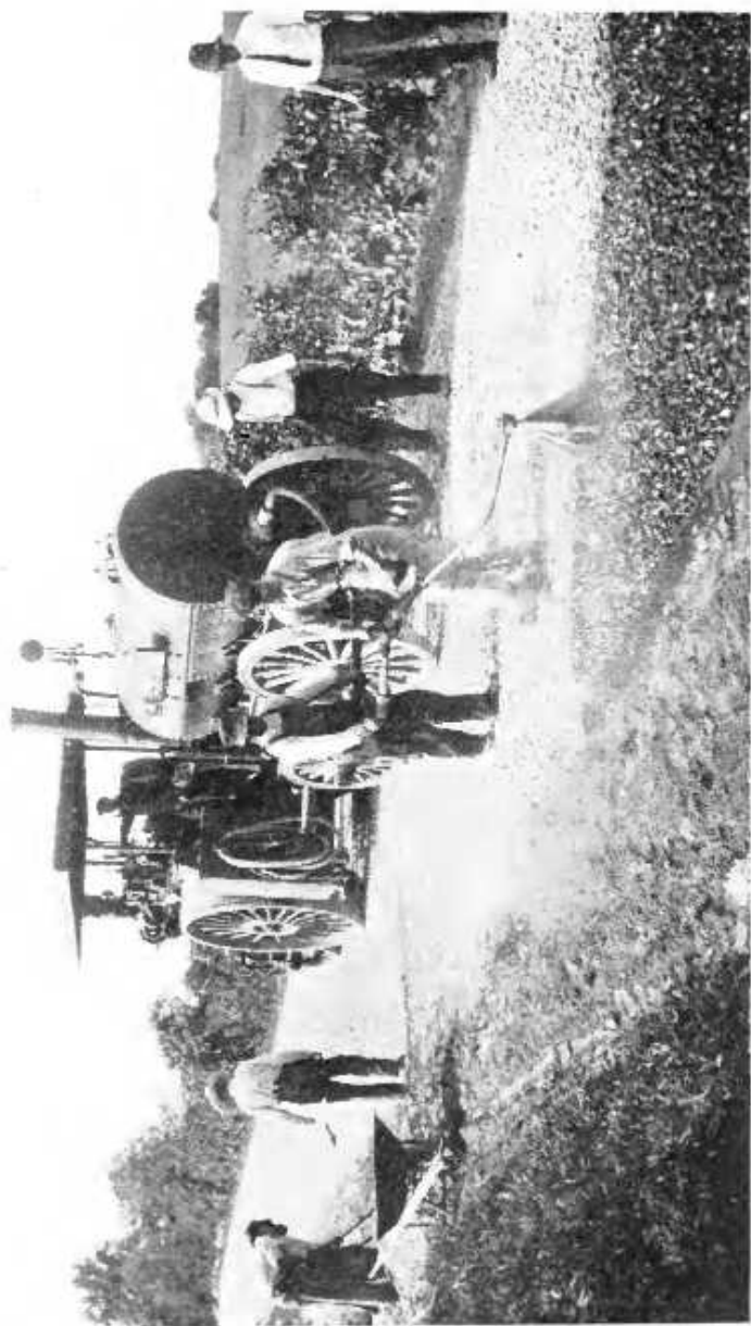
DISTRIBUTING TAR VIA COATING ON THE WEARING COURSE OF A SURFACED MACADAM ROAD Courtesy of Barrett Asphaltum Manufacturing Company, New York City
