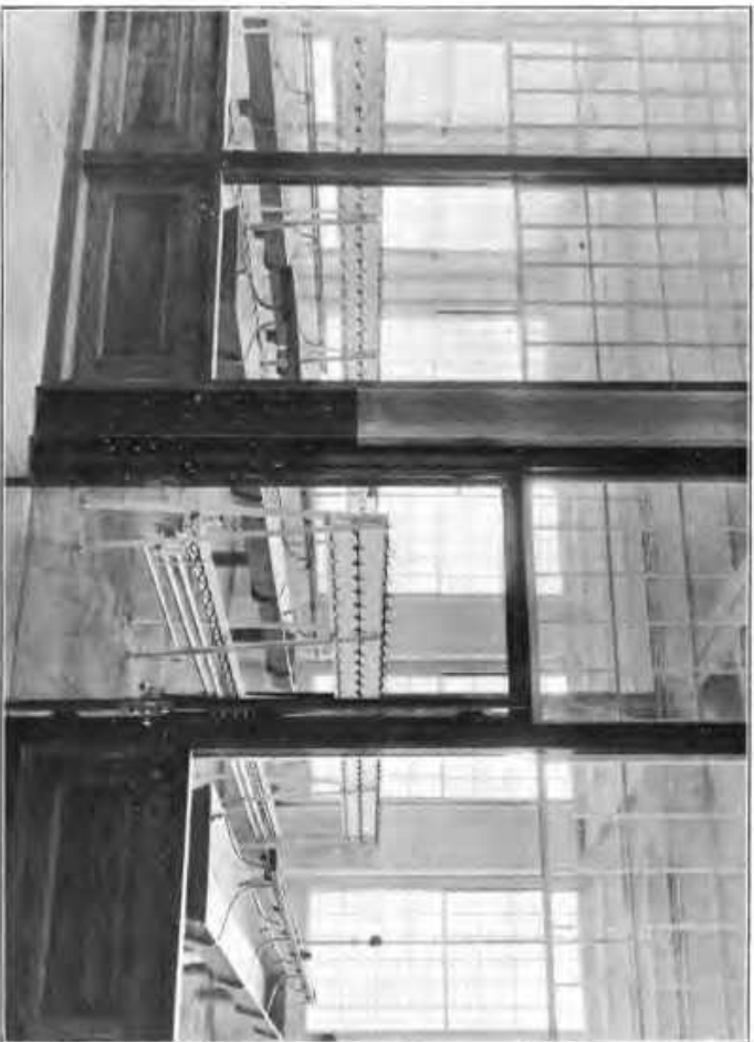
Wash Room in Machine Shop of Brown & Sharpe, Providence, showing arrangement for drying the outer garments of the workmen.
