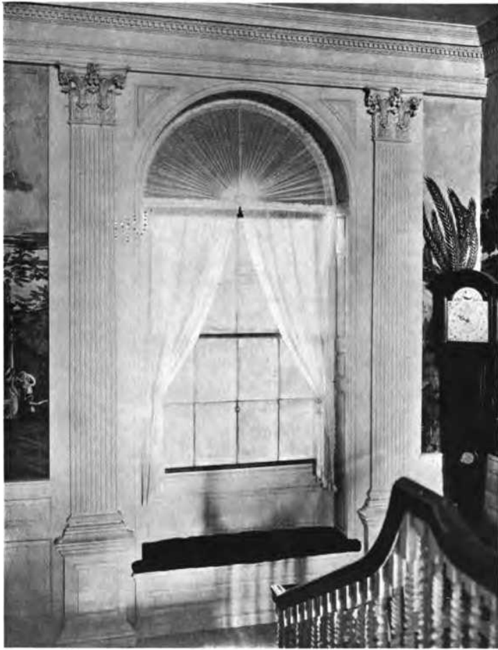
WINDOW ON STAIR LANDING, "THE LINDENS," DANVERS, MASS. BUILT IN 1770
