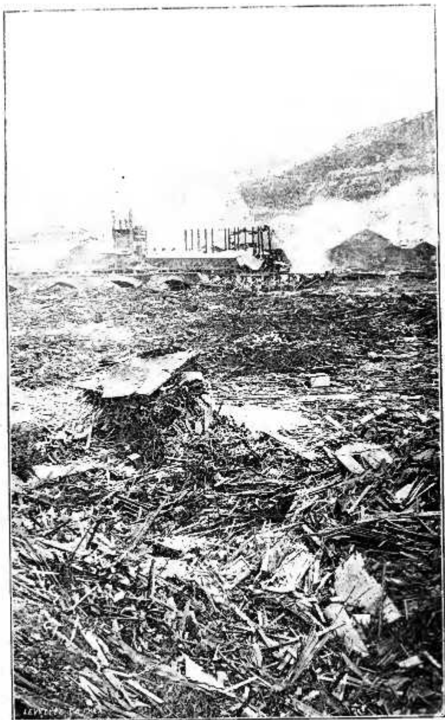
THE FIRE TRAP AT THE STONE BRIDGE.
